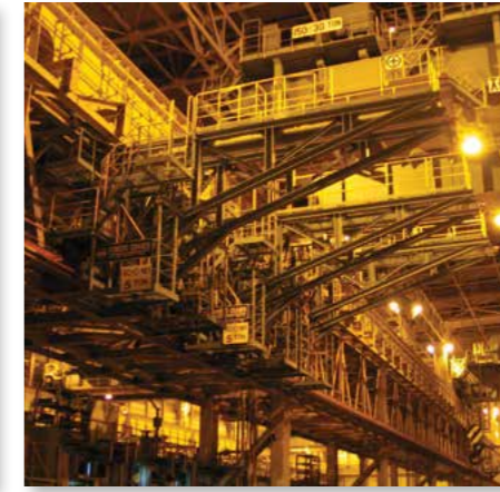
Wall Jib Hoist Crane
