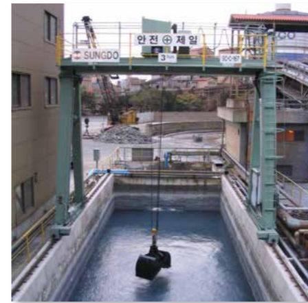
Bucket Hoist Crane
