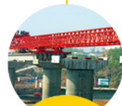
架桥机 Bridge erecting machine
